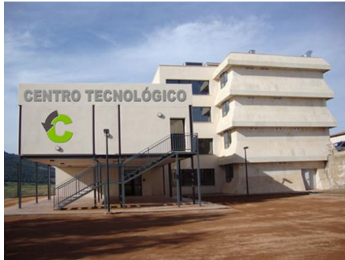
MERCURY TECHNOLOGICAL CENTRE Cerro San Teodoro s/n 13400 ALMADEN (Ciudad Real)
